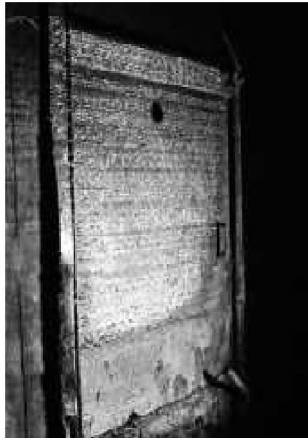
7. and 8. Corroded communications installation and metal door inside of the Goebbels bunker.
