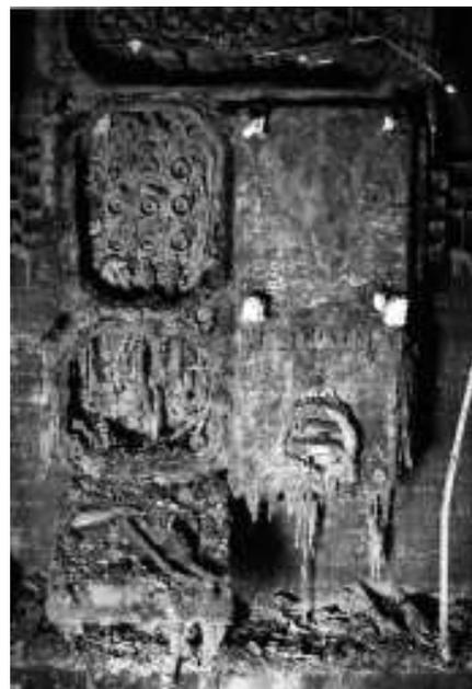
9. and 10. Goebbels bunker: light switches and corroded electrical installations.
